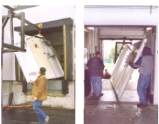
Walls of "knockdown" building are maneuvered through door measuring 7-foot square.
