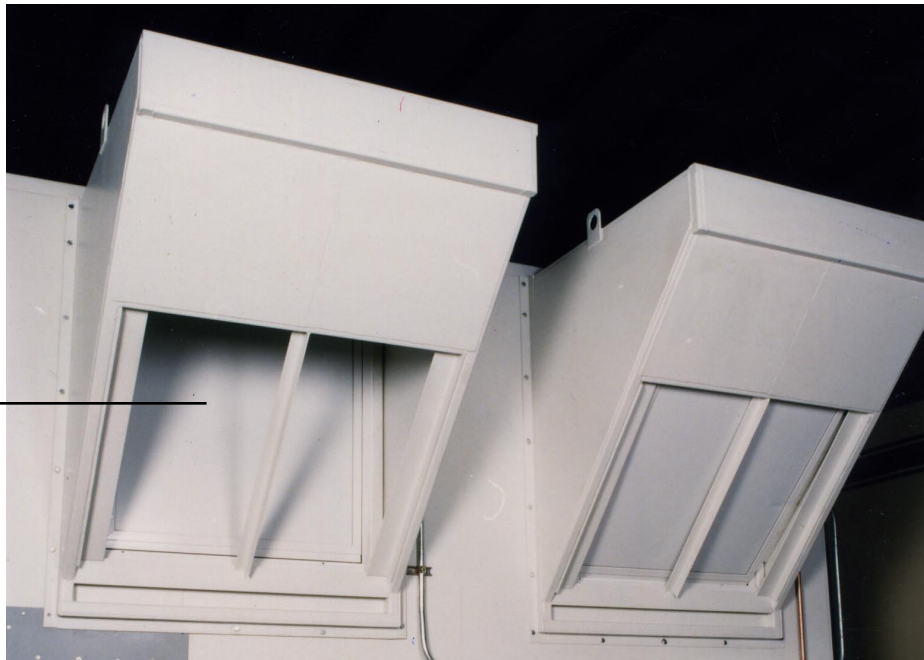
Patented blast shafts enable buildings to be placed close to existing facilities.
