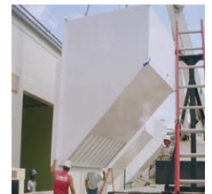
Patented blast shafts enable buildings to be placed close to existing facilities.
